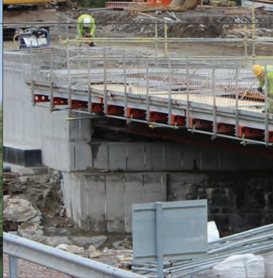
The new Allt Chonoglais bridge under construction △
