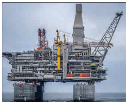
▽ Stainless steel fire and blast walls were installed on the Arkutun Dagi platform
