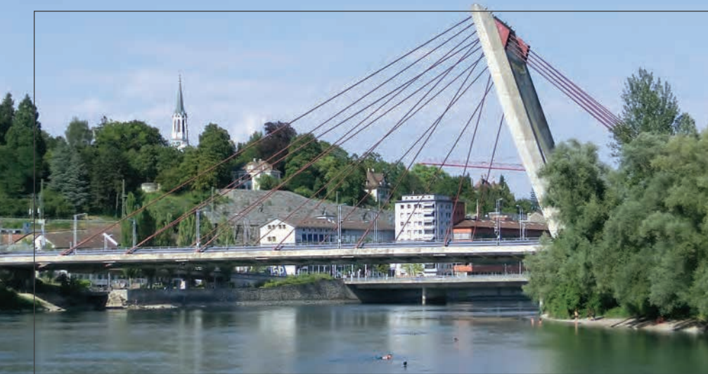
△ Schaffhausen Bridge was designed with an 80 year lifespan
