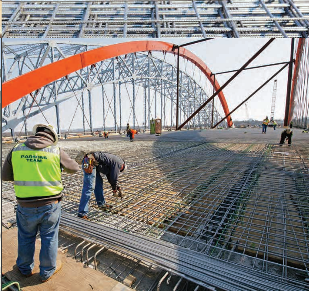
△ Alloy 2304 stainless steel rebar for the Hastings Bridge, Minnesota, USA project supplied by Contractors Materials Company
